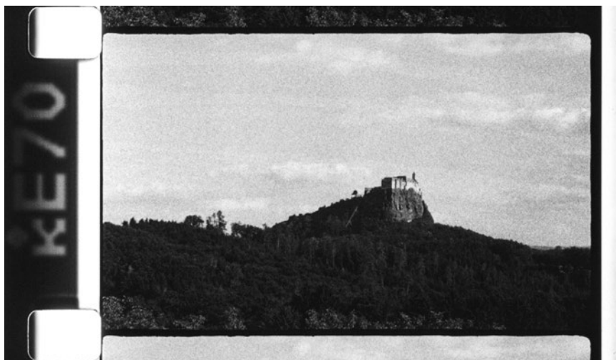
[One Channel of the 9-channel AV-installation Riegersburg ]
